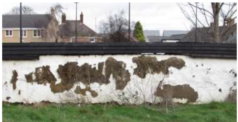
Scaffolding and deteriorating mud walls
