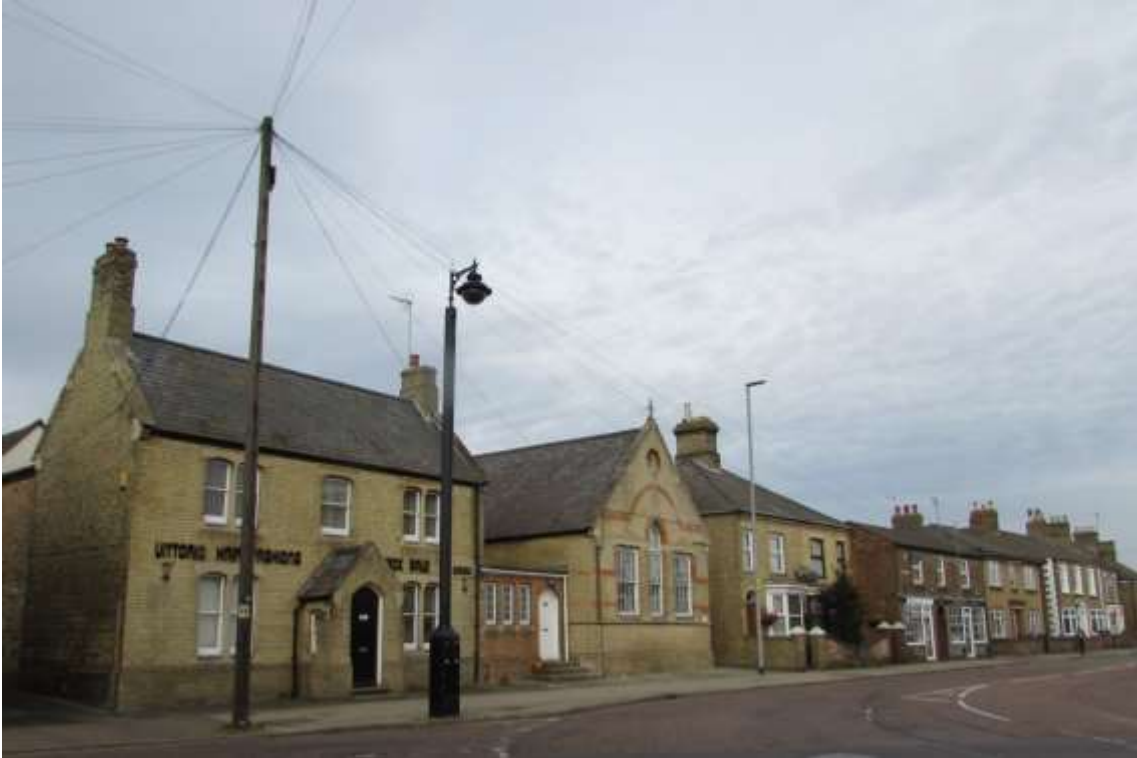
The 19 th Century former school building now a commercial premises and flats has a noticeable presence in the Broad Street scene
